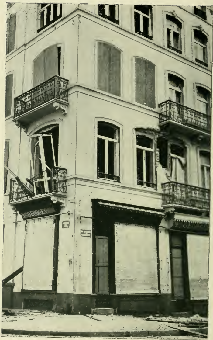
A "DIRECT HIT" ON A HOUSE NEAR THE HOTEL LITTORAL
