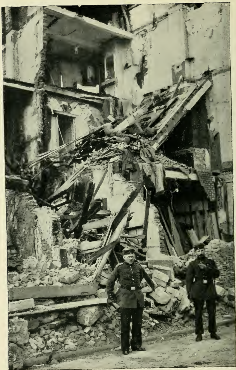
A HOUSE OF MALINES "LAID OPEN" BY SHELL FIRE
