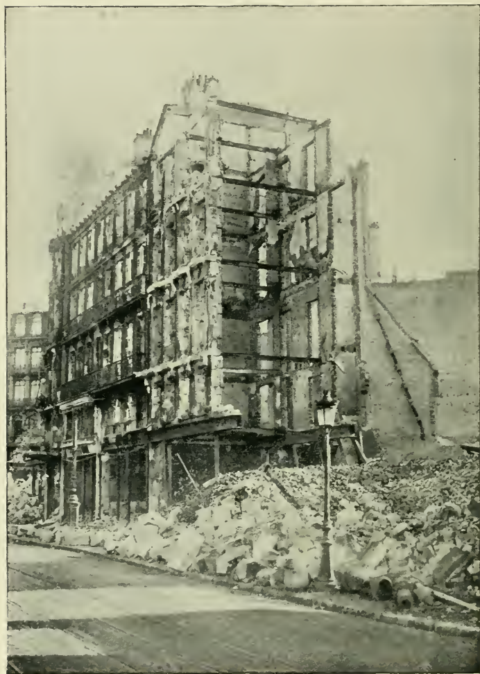
OF SOME HOUSES THERE IS ONLY THE SKELETON LEFT
